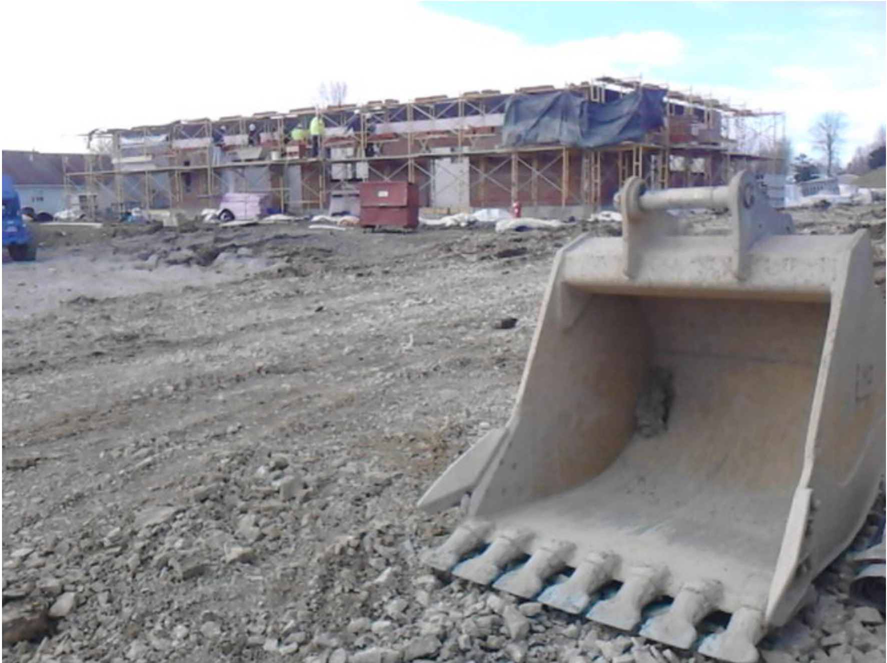
March - Water treatment plant
